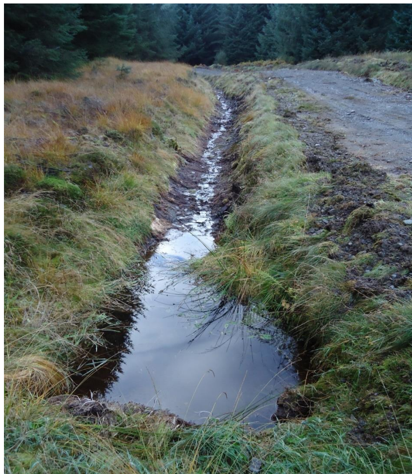
Plate 13.2: Typical existing access tracks and associated drainage
