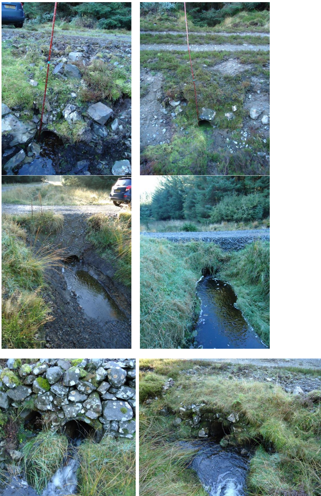
Plate 13.6: Existing culverts at the site
